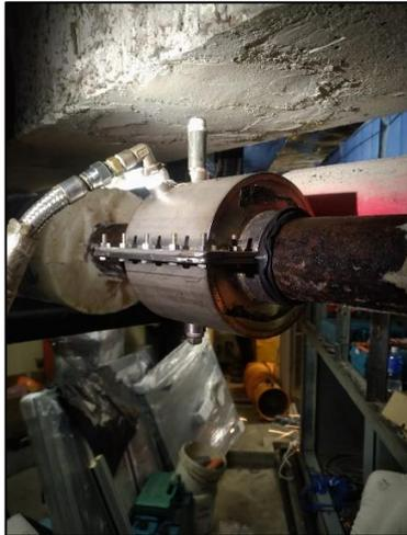
Installation of pipe freezing jacket at proposed location
